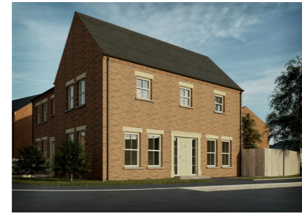
Style G1 3 Bedroom Semi-Detached Site Nos: 63, 67
